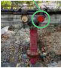
SE has already replaced a new valve cap.
